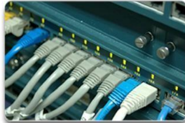
Cables must be connected correctly.
